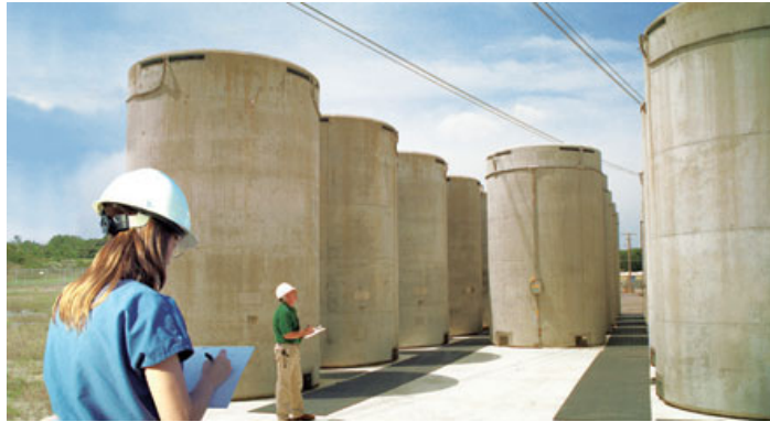
Figure 3. Dry casks containing spent nuclear fuel are inspected at an unspecified U.S. nuclear power plant. The cask design includes radiation shielding, so that approaching and handling these casks exposes the workers to a negligibly low radiation dose. (source: Nuclear Energy Institute)
