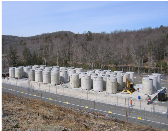
Figure 1. Spent nuclear fuel in dry casks is shown here at the Connecticut Yankee nuclear power plant site. This storage area is all that is left of the now-decommissioned nuclear plant, which generated 580 MW of electricity for 21 effective full-power years. (source: http://www.connyankee.com/html/fuel_storage.html )
