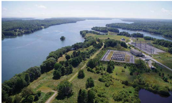
Figure 2. The site of the now-decommissioned Maine Yankee nuclear power plant. The site has been returned to “green field” conditions with the exception of the spent fuel dry casks, which are stored in open air within the small well-fenced area shown in this picture. (source: Bangor Daily News)
