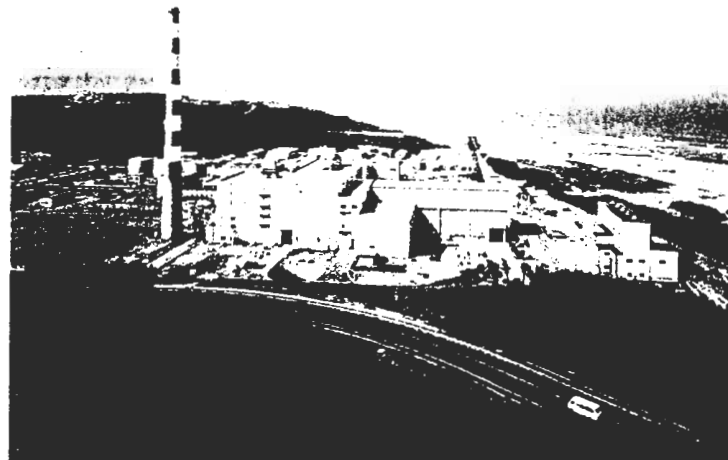
Fig. 13. PNC reprocessing plant at Tokai Works, Japan.
