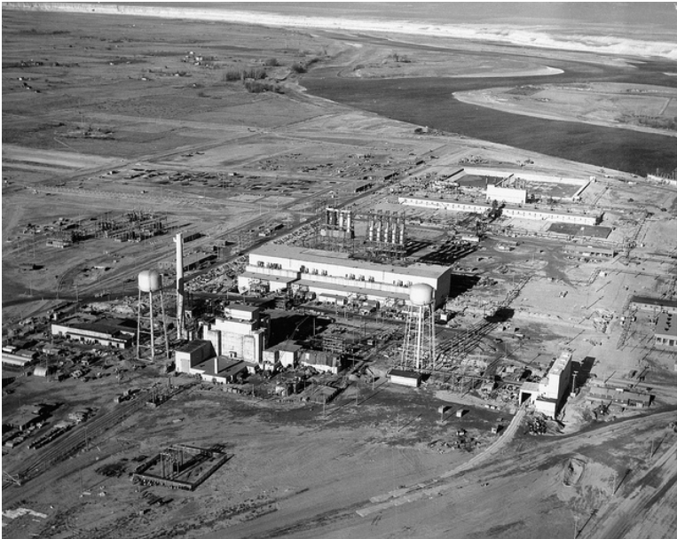
F Reactor complex at Hanford under construction, ca. 1944. Image is in the public domain.
